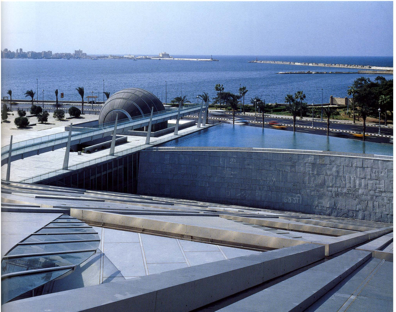
120 Sandwichmodule bilden die Dachfläche (o.); Angelagertes Planetarium (u.) | The roof surface is comprised of 120 modular sandwich panels (above); adjacent planetarium (below)
