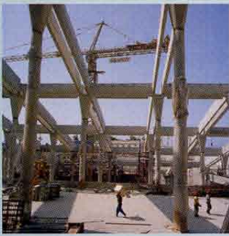
SUPPORT MORE THAN 400 PRECAST 46-FOOT-BY-6-FOOT-BY-1-FOOT ROOF BEAMS, WEIGHING AS MUCH AS 18 TONS. THE ROOF, ANGLED AT 16.08 DEGREES FOR OPTIMUM SOLAR SHADING, COMPRISES BAYS FILLED WITH ALUMINUM PANELS SANDWICHING AN ALUMINUM HONEYCOMB. ALUMINUM-WRAPPED, STEEL-
