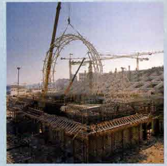
FRAMED MONITORS IN MANY OF THE BAYS ELIMINATE THE NEED FOR ARTIFICIAL DAYLIGHTING IN THE READING ROOM. THE PLANETARIUM IS CONSTRUCTED OF SIX PREFABRICATED STEEL TUBE TRUSSES WELDED TOGETHER, LIFTED INTO PLACE ON SITE, AND LATER WRAPPED IN GRP PANELS.
