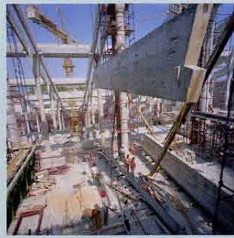
SUPPORT MORE THAN 400 PRECAST 46-FOOT-BY-6-FOOT-BY-1-FOOT ROOF BEAMS, WEIGHING AS MUCH AS 18 TONS. THE ROOF, ANGLED AT 16.08 DEGREES FOR OPTIMUM SOLAR SHADING, COMPRISES BAYS FILLED WITH ALUMINUM PANELS SANDWICHING AN ALUMINUM HONEYCOMB. ALUMINUM-WRAPPED, STEEL-
